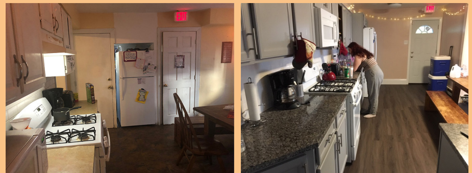
The TLC kitchen, before (left) and after the renovation.
